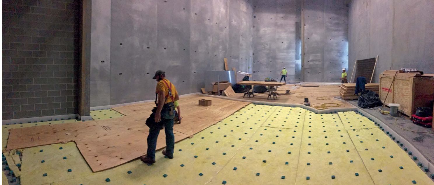
The room layout begins to take shape as the floating floors are laid down.
