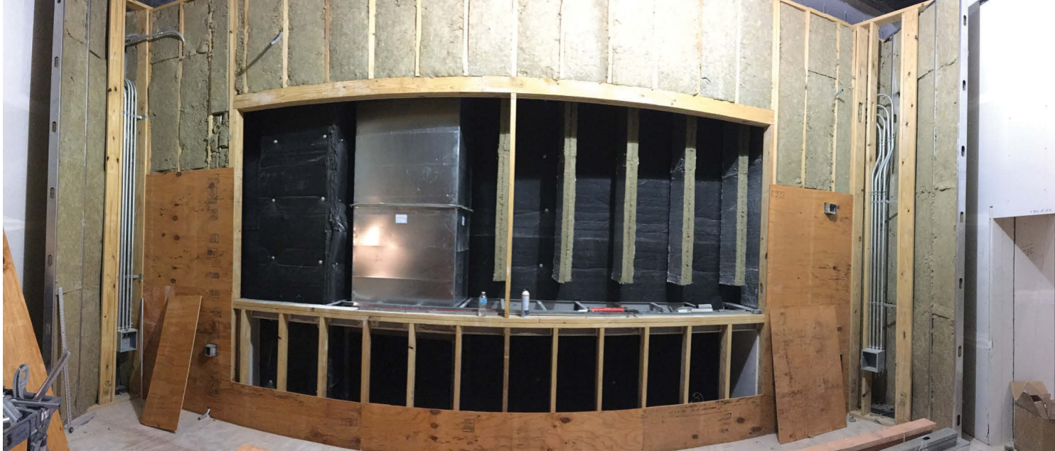
The wall-within-wall construction of the live room, which allows for HVAC returns and 4-inch hanging batts for trapping low end that enters from the open space at the top of the inside wall.
